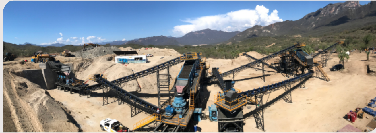
150 t/h Plant, Mexico
