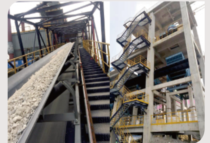
Lafarge Cement 500 t/h Project, Sichuan, China
