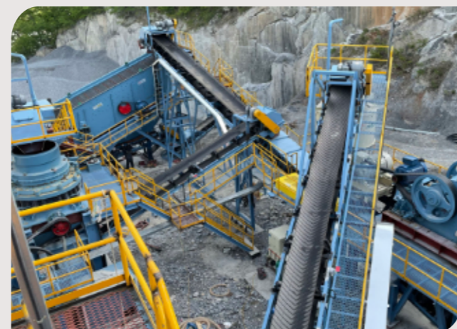
230 t/h SYSTEM Plant, South Korea
