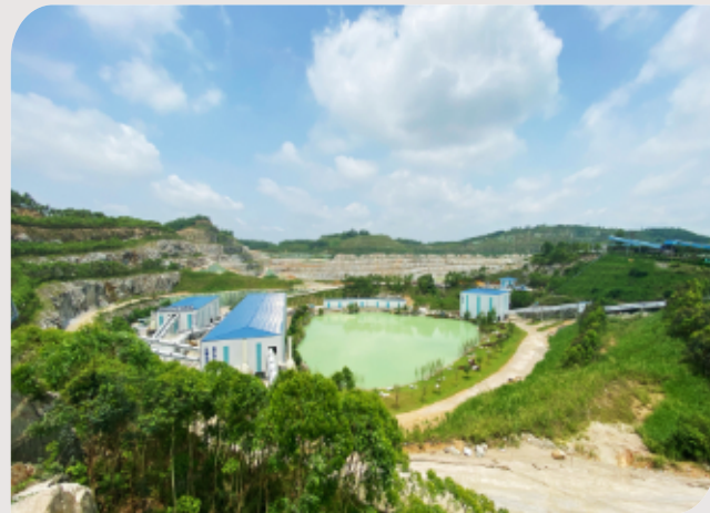
Sand-making Line with 3 million ton annual output, Guangdong, China
