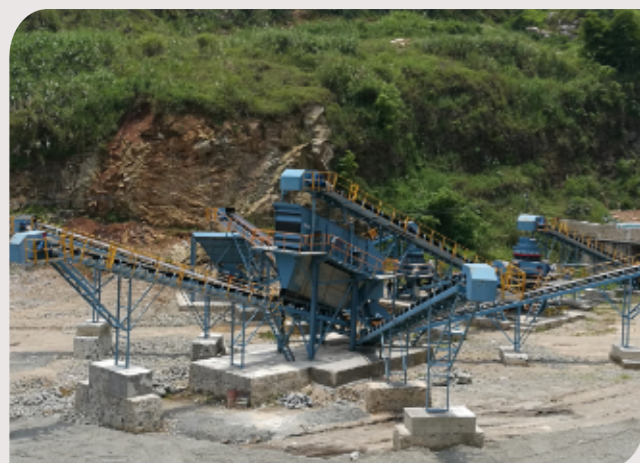
250 t/h SYSTEM Plant, Lembang, Jawa Barat, Indonesia
