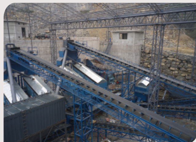
500 t/h Limestone Project, Wulong, Chongqing
