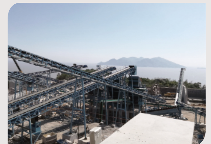
Nuclear Power EPC Project, Fujian, China
