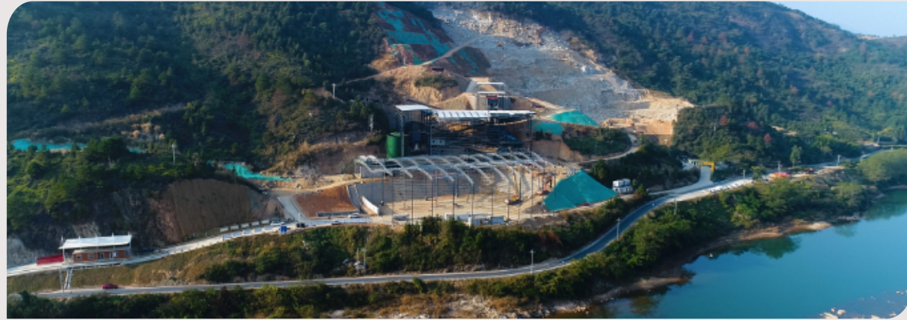
Xiashanwan Quarry 800 t/h Project, Jiangxi, China
