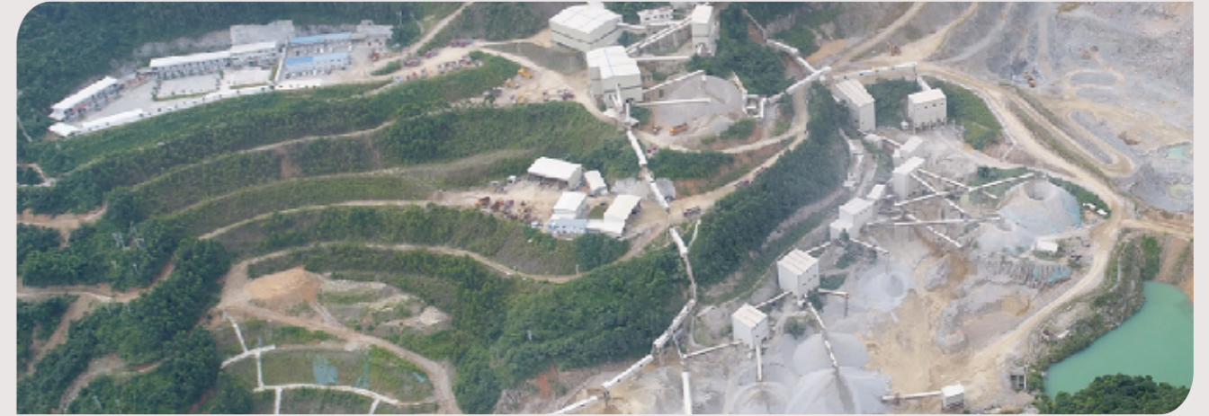
Yunfu Quarry, Huayue Group 1000 t/h+2*750 t/h Project, Guangdong, China
