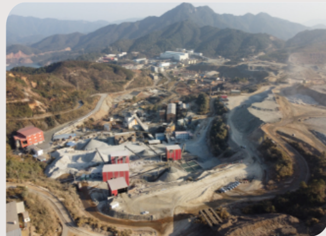
Dabaoshan Iron Mine 1000 t/h Project, Guangdong, China
