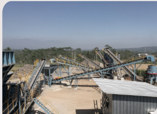
150 t/h Aggregate Plant, Subang, Indonesia
