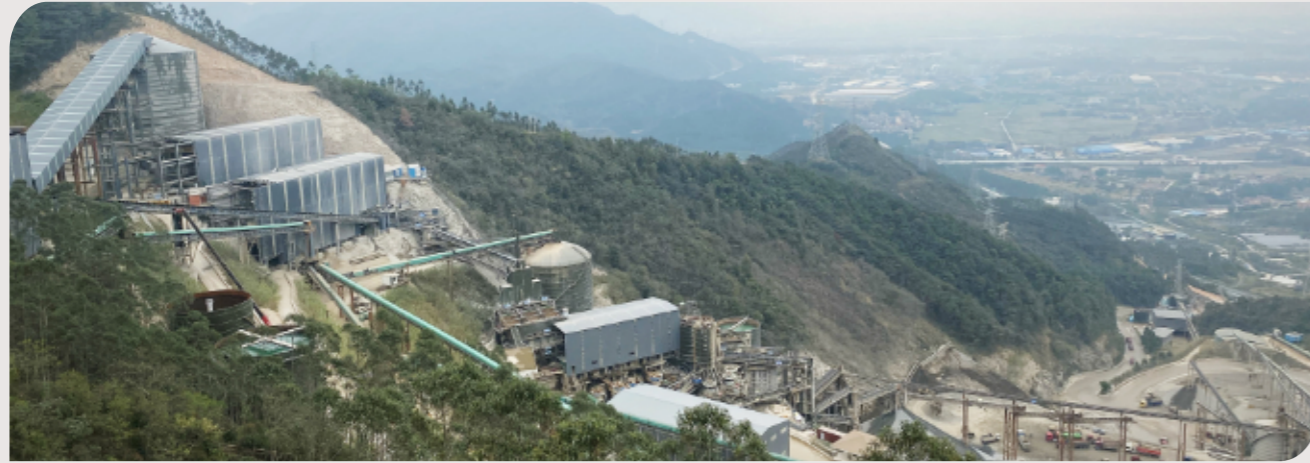
Gucheng Group 9×SCH8000,3500 t/h Project, Guangdong, China
